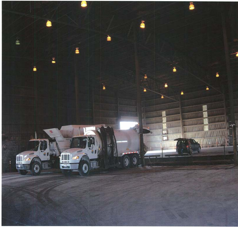
Exhibit 9. Environmental Excellence Transfer Station
